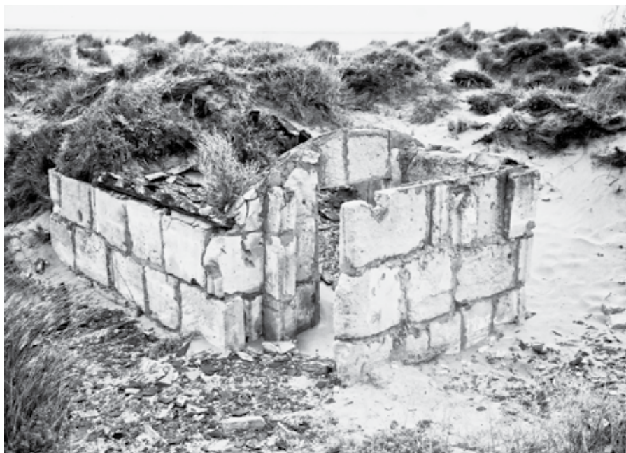
Figure 1 Remains of German military defenses in the Réserve Nationale de Camargue near the Phare de la Gacholle (March 2005). © Chris Pearson
